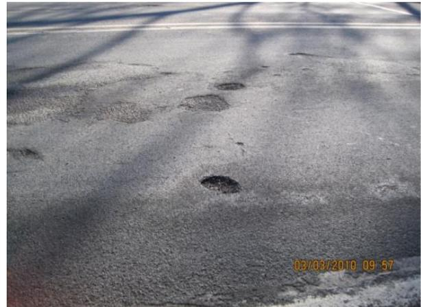
**Appendix A, Figure 15. Stripping of asphalt pavement caused by water damage (State of Minnesota Department of Transportation, 2010)**
